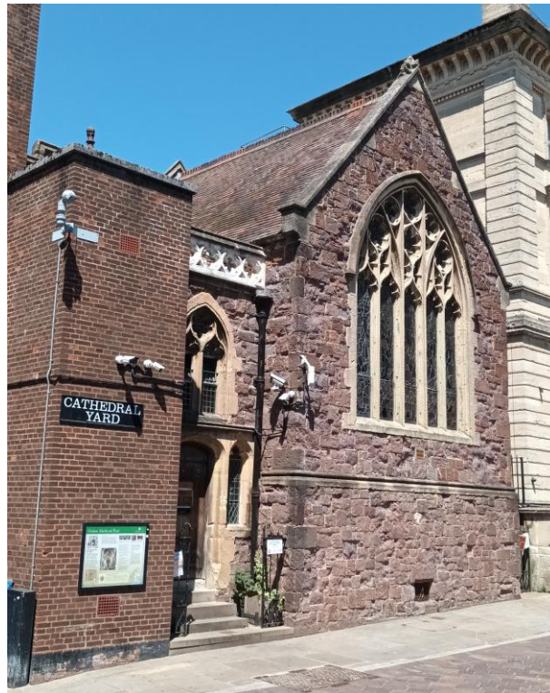
St Petrock's Centre in Cathedral Green
